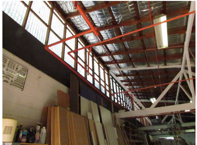
Polycarbonate clerestorey and exposed roof framing in the rear unit
