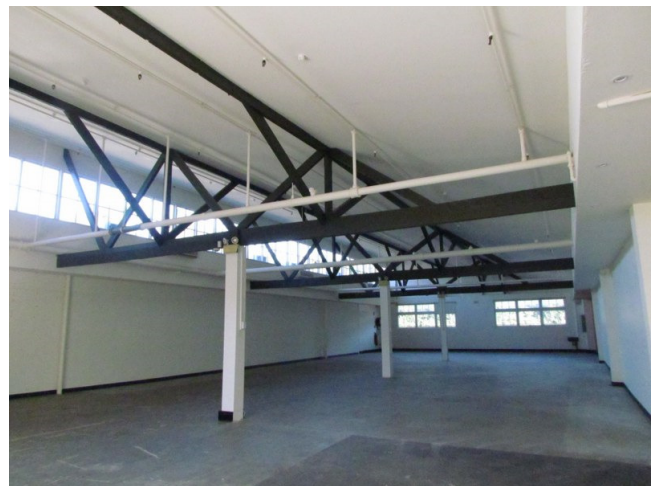
Upper floor level unit, looking west. Side dividing walls are a later addition.
