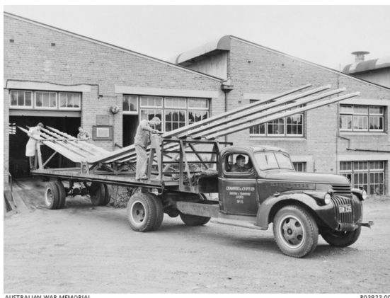
Employees of F Dickin Ltd loading the rear spar for transport c.1945. Milton Kent photographer. (Australian War Memorial)
